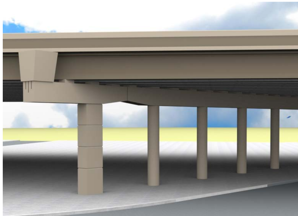
Widening where decorative column is not possible provide extended Cap, Cap Ear Wall and decorative column - Skewed bent location
